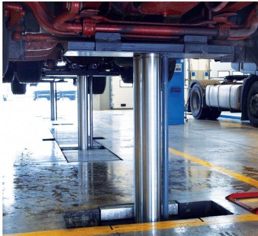
All SLiFT TRUCKLIFT systems have synchronization control based on DIN EN 1493.
