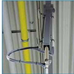
The E-BOX is attached to the ceiling or mounted to an on-site profile using a special fastening set.
